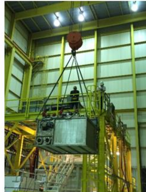
Confirmation of fit-up and functionality of production equipment
